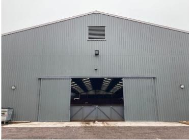
Picture Three: An example of additional ventilation hatches (this building has seven spread around the building on each wall) to ensure high ACPH
